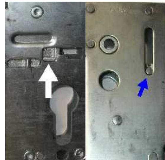
**LH side:** Locate hole already in case 140mm up, (red arrow). To the left you will see a plate with a small hole in it (yellow arrow) angle small screw driver in and lift the plate approx 10mm after which you should then see a V notch in the plate. Lift the plate as high as possible to complete the retraction of the mechanism. If you cannot get a tool onto the plate then drill a hole approx 10 mm fwd, inside the handle profile.
